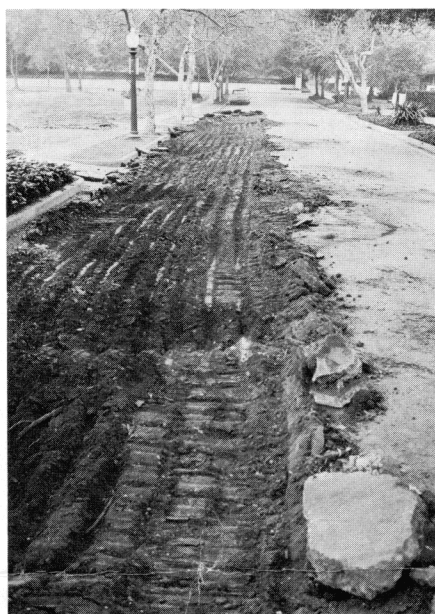
ABOVE —The beginning of the end for Mentoria Court.
